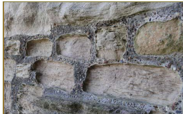
The application of inappropriate mortar causes damage to natural stone walling.
