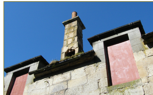
Heavy vegetation growth caused blockages to rain water goods.
