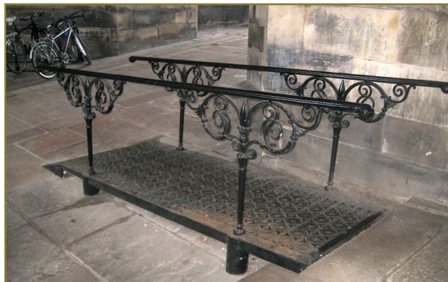
Temporary ramps avoid disruption to historic fabric. © Courtesy of Historic Environment Scotland.
