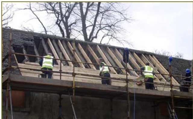
Installation of replacement roof timbers .
