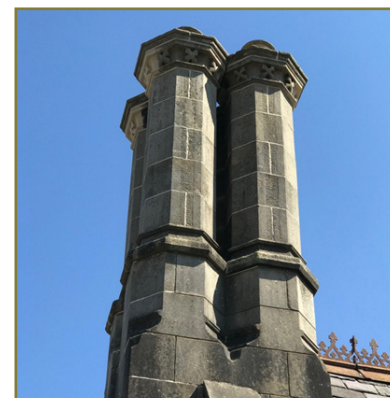
Chimney stacks reinstatement following roof repairs.
