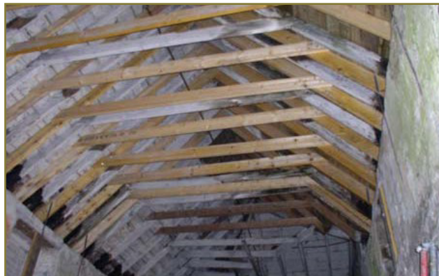
Interior of the Stables with new roof trusses in place.
